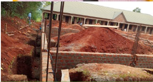
Halted progress of new school building. The hope is to take children from Primary to Secondary School.
